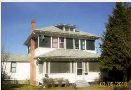
250 Leathead Road $5,000 (new roof, paint and gutters)
