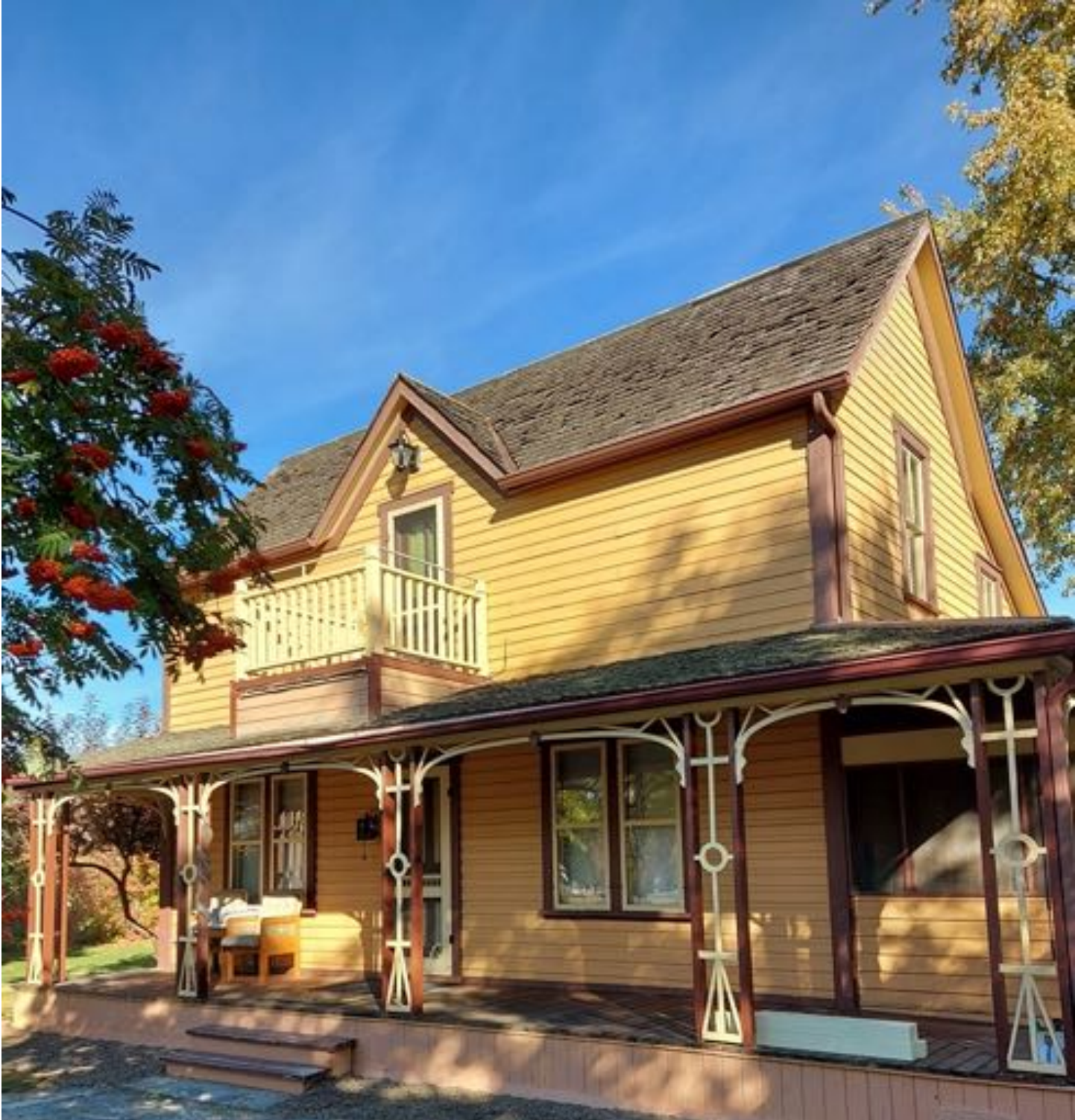
Mclver House - home to our building and property caretaker
